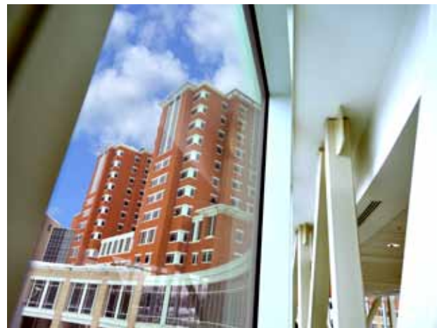
View of the new pavilion from the concourse bridge
